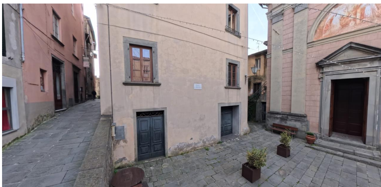
Figure 26 exterior of the Church of S. Annunziata and access door
