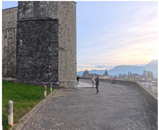
Figure 21 back of the Cathedral and terrace
